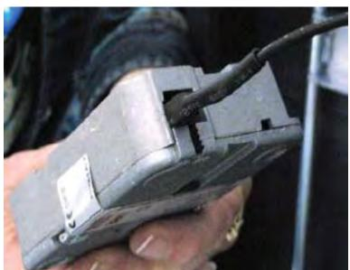
Push the excess cable carefully back into the door opening.
