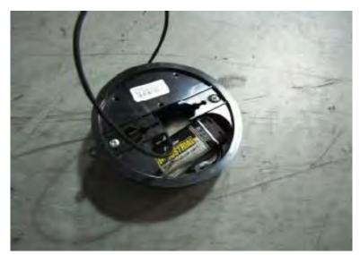
From the outside of the door, feed the data cable through the opening between the two bolts. Push all of the cable into the cabinet.
