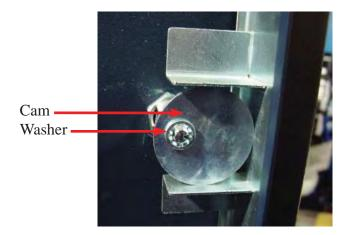
7. Ensure all hardware is tight. Test the lock before closing the door. Observe that the key can only be removed when the door is locked. (Key horizontal)
