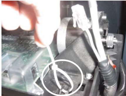
Cable tie wrap near data / power connections.
