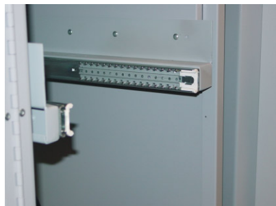
Figure 5. Push the rails into the cabinet before installing the dispensing mechanism into the cabinet
