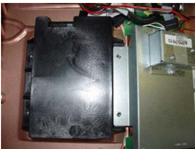
Figure 9. Install EPP device.
