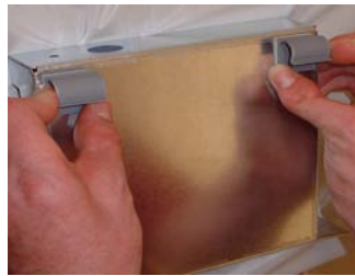
Figure 2-34. Affix cable clips.
