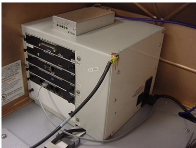
Figure 2-17. RS-232 cable routed.
