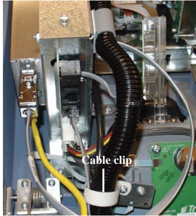
Figure 2-37. External Ethernet cables routed and connected.
