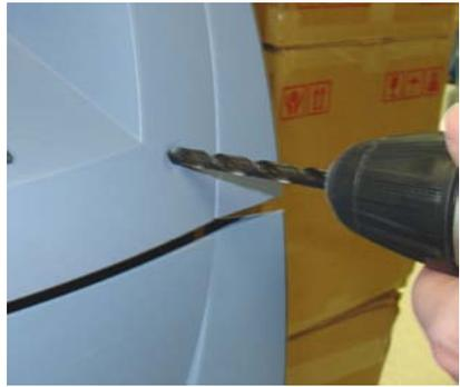
3. Clean/smooth any burrs or rough edges on the inside and back of the hole. Vacuum or brush any shavings on the inside of control panel.
