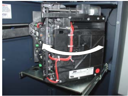
Rotate mechanism to “Service” position (clockwise).
