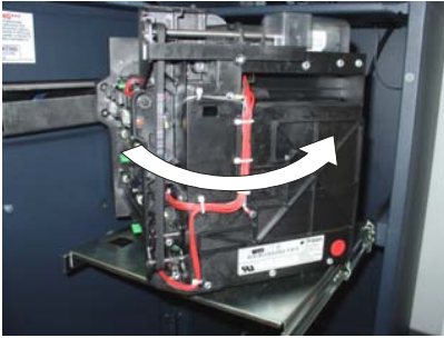
Rotate mechanism to operate position (counterclockwise).
