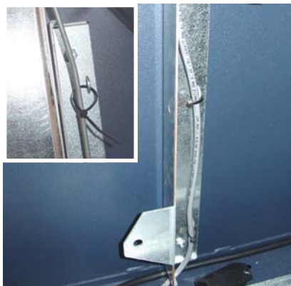
Figure 7. Route power cable behind bracket and secure with ty wraps.
