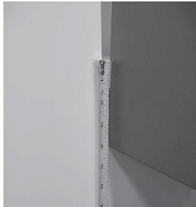
Figure 2. Measure from bottom of wall opening to bottom of sleeve.
