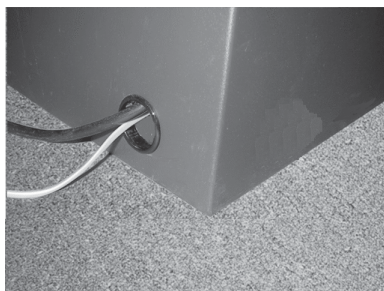
Figure 2. Install snap bushing on access hole that carries power and phone cords.
