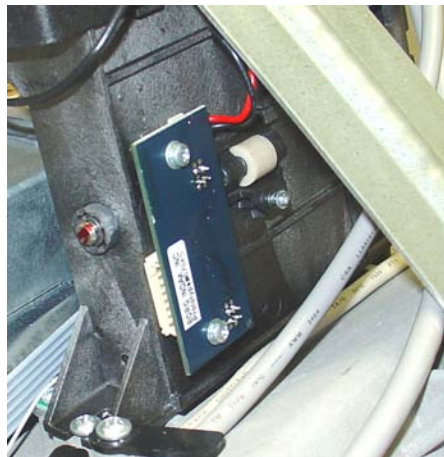
New presenter board installed.
