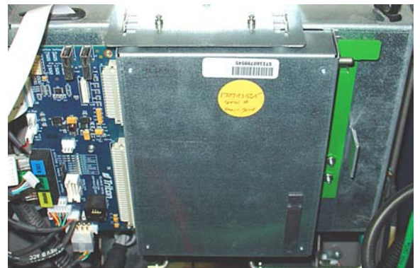
X2 main board installed.
