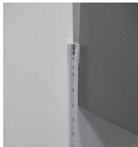
Measure from bottom of wall opening to bottom of sleeve.
