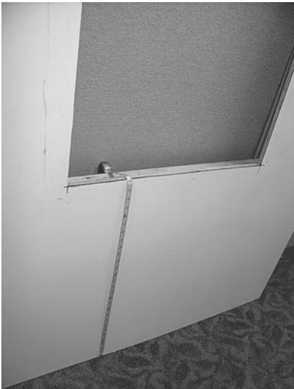
Figure 1. Determine height of opening to inside floor.
