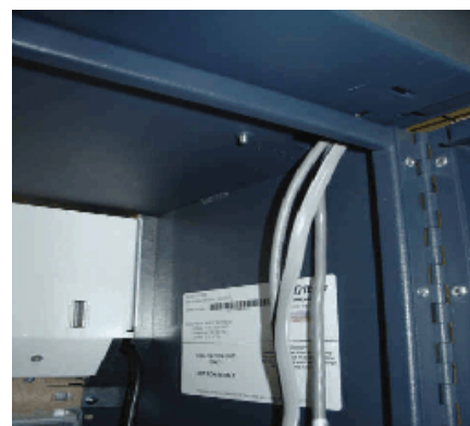
Figure 5. View of cables from inside sleeve cabinet.
