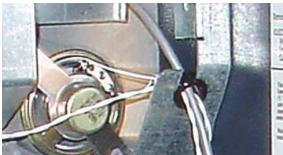
Route cables through grommet.
