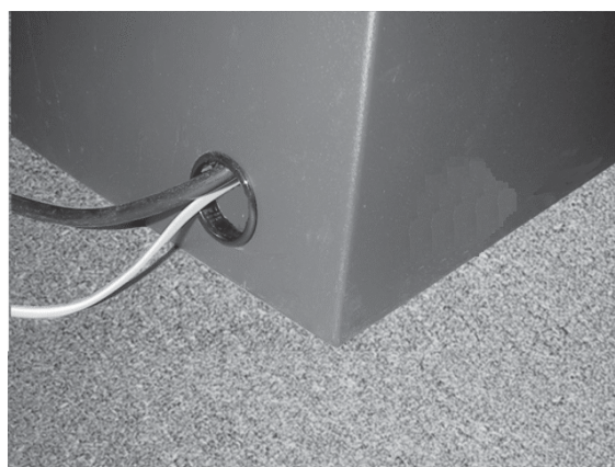
Install snap bushing on access hole that carries power and phone cords.
