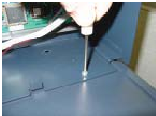
Figure 6. Secure RSP to top of cabinet.
