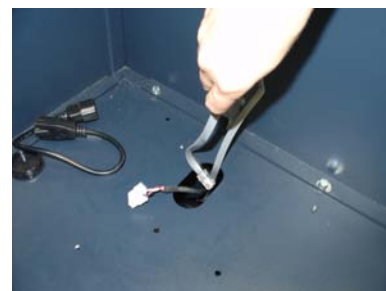
Figure 5. Feed cables down to vault area.
