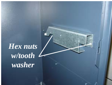
Figure 11. Side rails removed.
