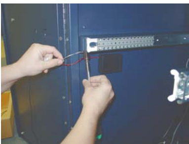
Figure 10. Remove door ground bolt.
