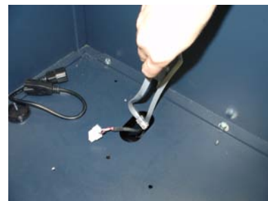
Figure 5. Feed cables down to vault area.
