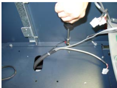
Figure 3. Disconnect ground wire.
