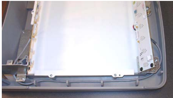
Jumper cable connected and routed.
