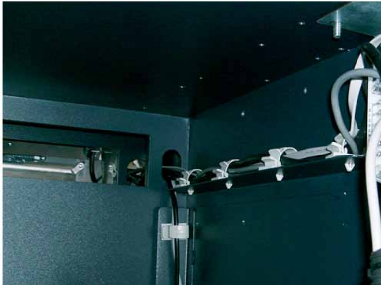
Right side cable routing to upper cabinet.
