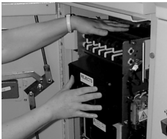
Figure 4-11. Installing the Reject Box.
