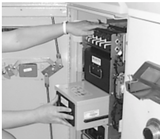
Figure 4-8. Installing a cassette.
