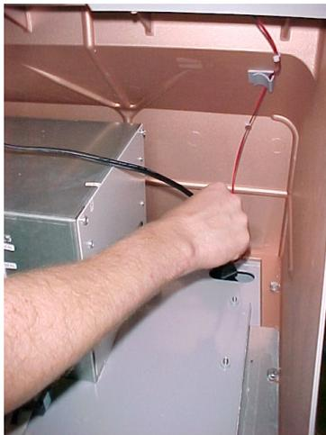
**Figure 2. Feed cable through access hole in top of vault.**
