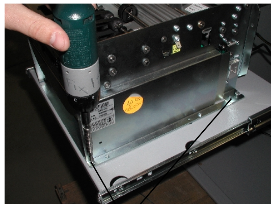
Attach the dispenser to the tray with two screws on each side.
