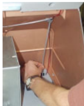
Figure 4-42. Route 4-Pin Modular Cable through cable access hole.
