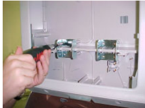
Figure 4-4. Securing Mounting Brackets.
