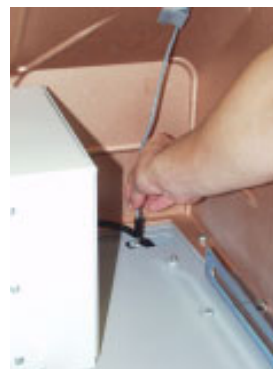
Figure 4-13. Feed Fan Power Cable into ATM security cabinet.
