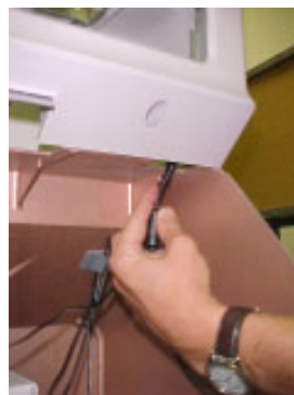
Figure 4-54. Feeding FMV Power Module cable into Hightopper enclosure.
